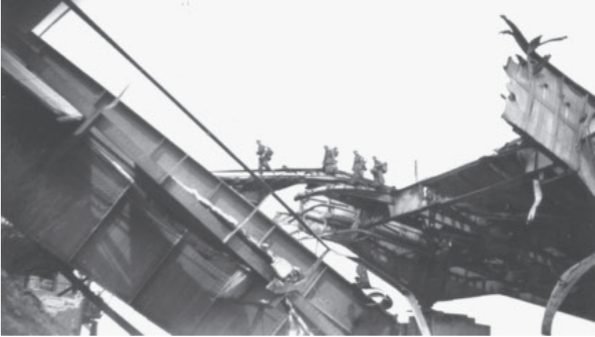
German soldiers crossing the Elbe River over the bombed-out bridge at Stendal.
